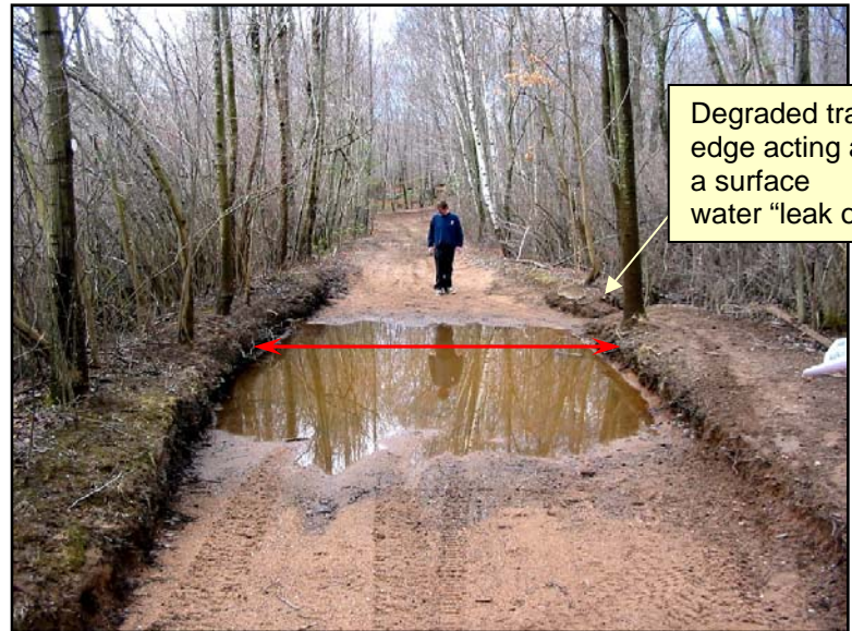
Photo 5. Chalker Brook passes through a culvert that is in need of improvement and repair. Seepage across the trail was observed suggesting either the culvert located in the vicinity of the red arrow is either undersized or is partially crushed or blocked.
