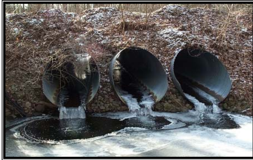
Figure 1. Culverts perched above the streambed block upstream fish passage within Cold Brook
