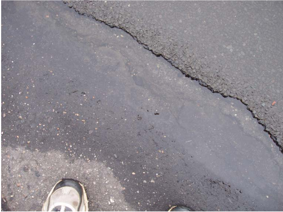
Many layers of asphalt.
