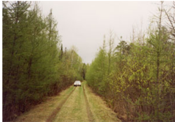
Figure 10—This road still maintains a free flow of water through the roadbed while providing a stable road surface.
