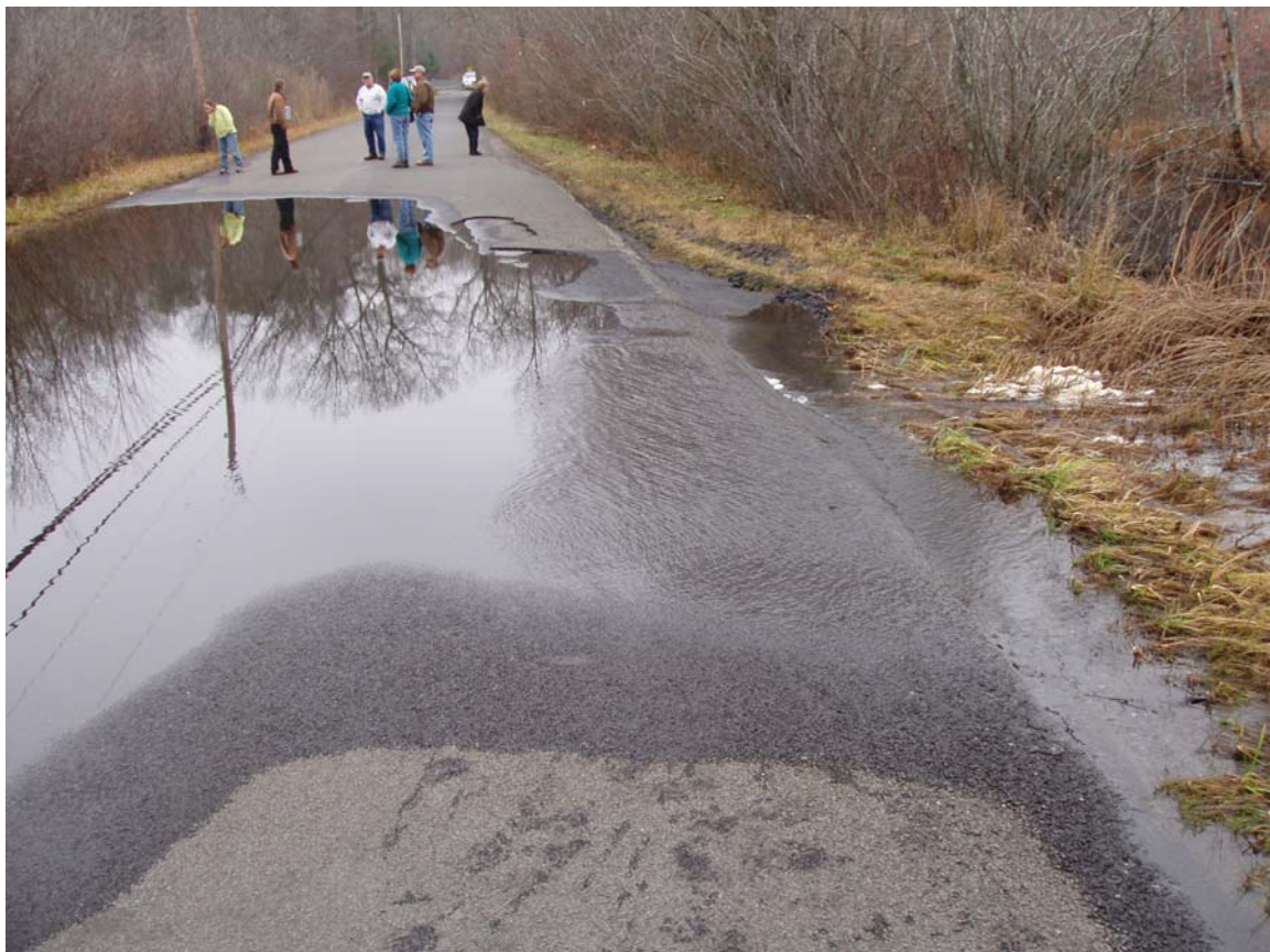
Water running over road surface in area of pipes under the road. (11/28/06)
