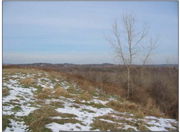
Top of the landfill looking north.
