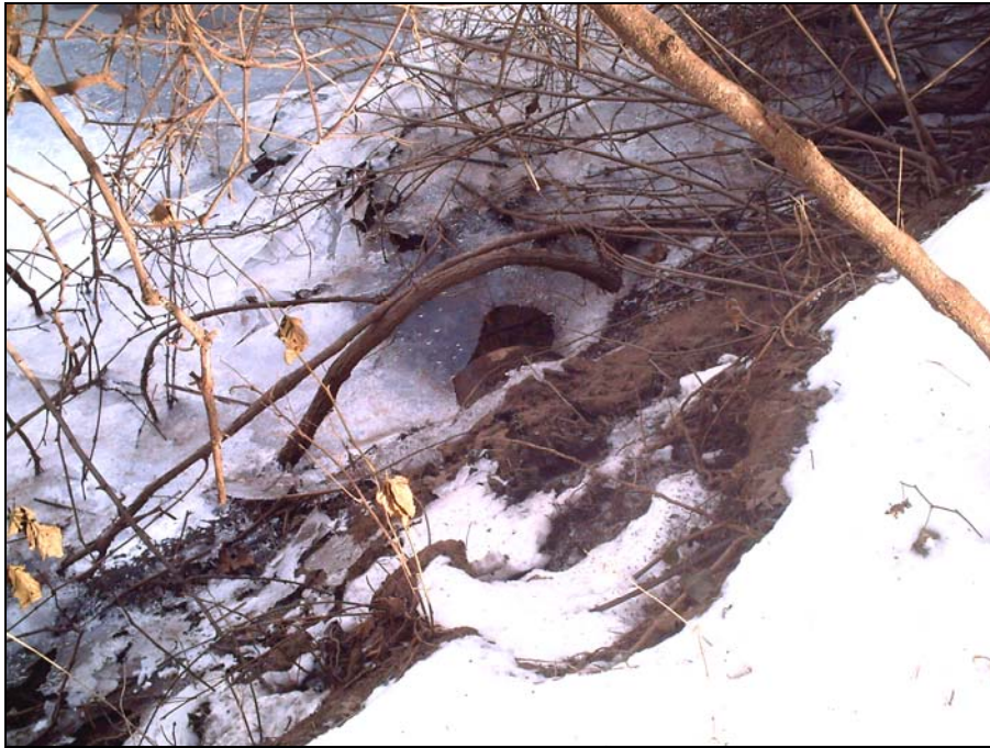
Figure 6 - this is a view looking down slope into the Mattabesset. Notice the 5 or 6 inches of concrete pipe emerging from the bottom of the bluff. The discharge from the pipe, though small, was constant and fell with sufficient energy to form a little plunge pool which kept the water open and ice free.
