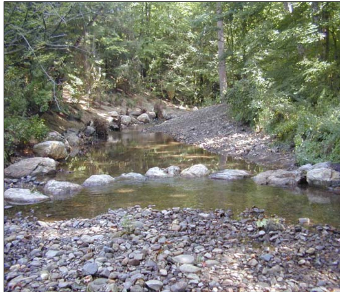
An example of a vortex rock weir.
