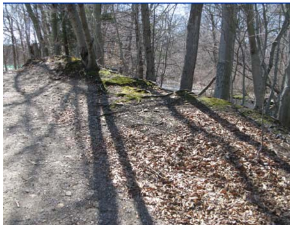
Figure 8. Artificial levee built to a height of 10± feet above flood stage. View taken near south central part of park near a wetland restoration area. Levee continues for about 1000 feet and ends abruptly in a swamp.
