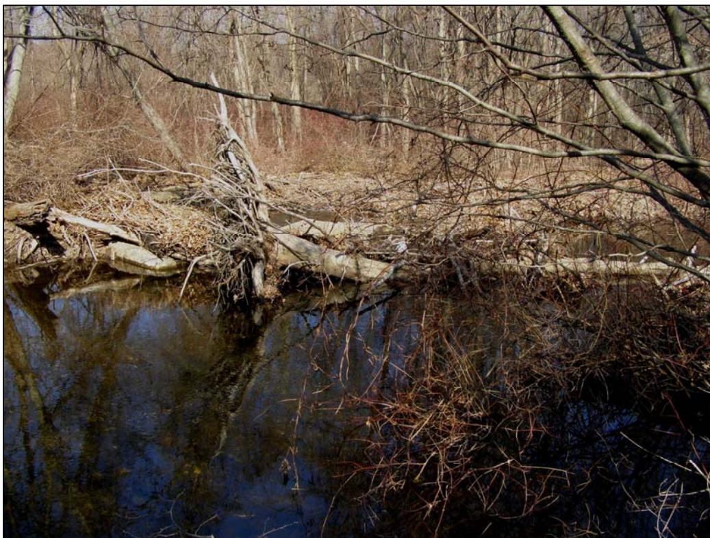
The diversion structure in the Wepawaug River. View of the structure is partially obstructed by fallen trees.
