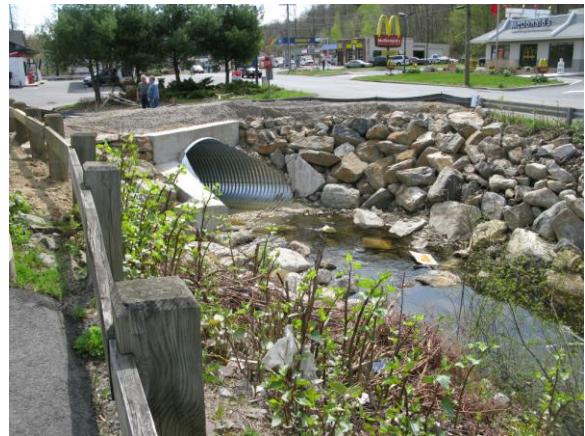
Figure 5. West entrance to mall on Rubber Avenue, looking downstream; bank on left. The conduit shown was replaced when a smaller conduit washed out during floods that accompanied precipitation of the remains of tropical storm Irene in August, 2011.
