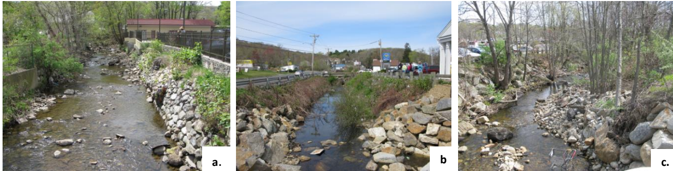
Figure 4. Floodplain encroachment. In all three pictures, fill has been placed to the very edge of the stream channel, eliminating the natural flood retention area. a. Looking upstream at Cherry Street crossing. The brook has effectively been channelized here. Regulating agencies even allowed building foundation to be installed on the stream bank. b. Crossing at west entrance to mall on Rubber Avenue, looking upstream; bank on right. Channelization has occurred here also, but the fill is not as high as at Cherry Street. The brook flooded here, in part because the channel is not as deep, but more importantly, the conduits below this crossing were sized too small. Here there is no floodplain, so in effect, when a heavy rain even occurs, the stream creates its own flood plain, spilling across the street and into adjacent buildings that are built where the flood plain was. c. Looking downstream at west entrance to mall. Regulatory agencies allowed filling of the floodplain up to the very edge of the river channel to create a parking area. Then the filled area was covered with an impervious surface.
