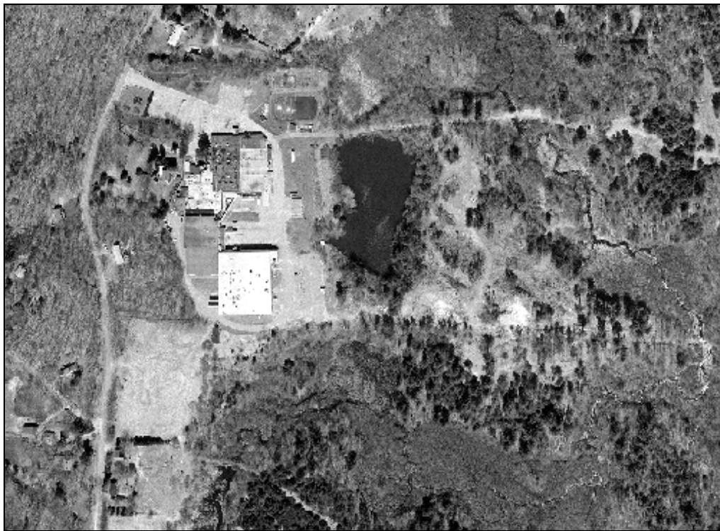
Figure 2 – The site in spring of 2004. The agricultural fields are long gone with tree, shrub and grass vegetation dominating the site. The pond has changed shape and, to the east, the course of the brook has changed. Agriculture probably ended in the late 1940s and revegetation of the site got underway.
