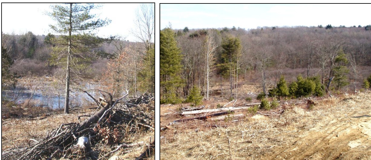
Figure 4 – Above are two views looking downslope and east into White Brook. In the left hand photo there is little vegetation between the bottom of the slope and the open water. Silt fence can be seen in the lower right hand corner. The final installation of silt fence will be backed by staked hay bales before excavation begins. In the right hand photo, in the lower right hand corner, bare dirt has been exposed on the downslope side leading to the wetland and there is no silt fence or erosion control of any kind in place. The vegetation on the flood plain of the brook is dominated by 15 to 20 foot high speckled alder ( Alnus spp. ).
