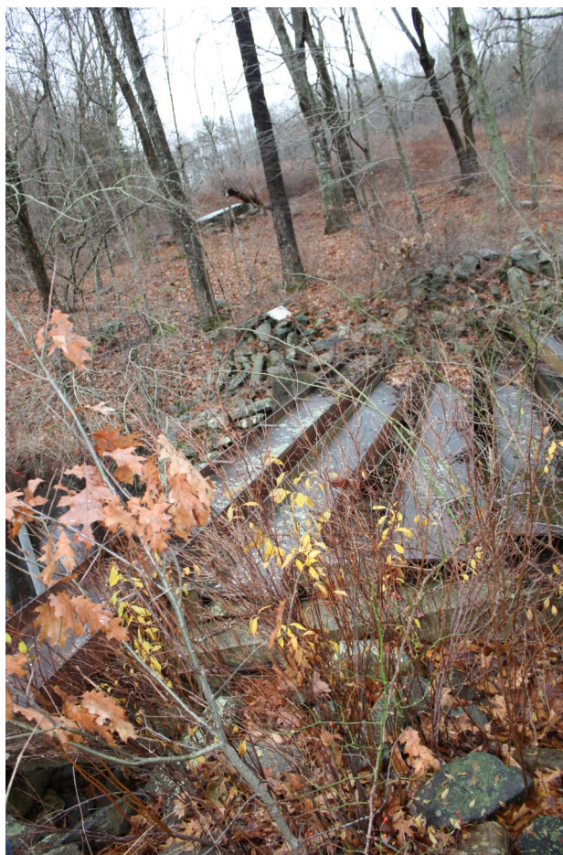
Figure A– 25– Photo of damaged Broadbrook crossing on south end near small dam. Source: J.Davies, CTC&D 2016
