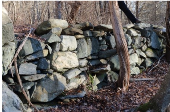
foundation wall with 3 flat, extruded steps" (3 rd step touches tree trunk)
