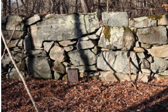
notebook at base of barn foundation is 13" tall
