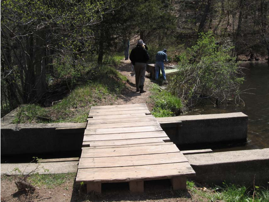
Outlet portion of corrugated metal pipes.
