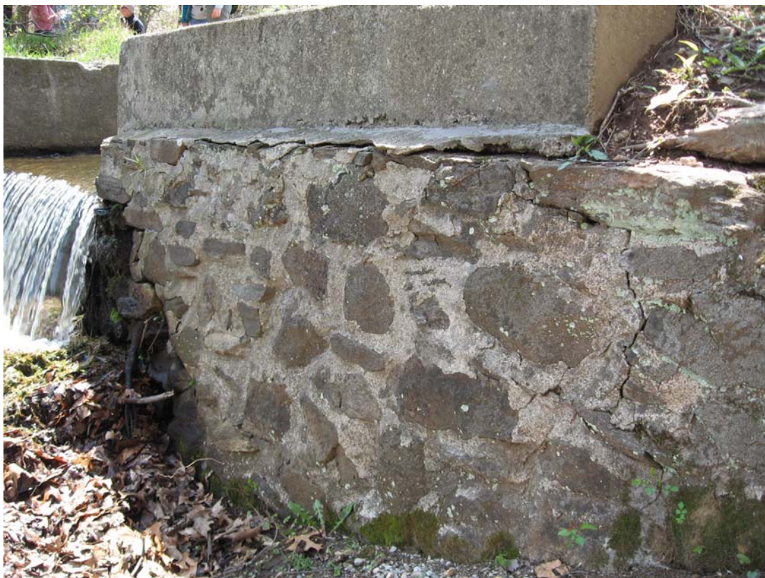
Downstream masonry wall with cracks and voids.
