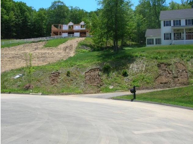
Slope Failure on Country Woods Lane
