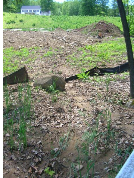
Silt Barrier Failure on Country Woods Lane
