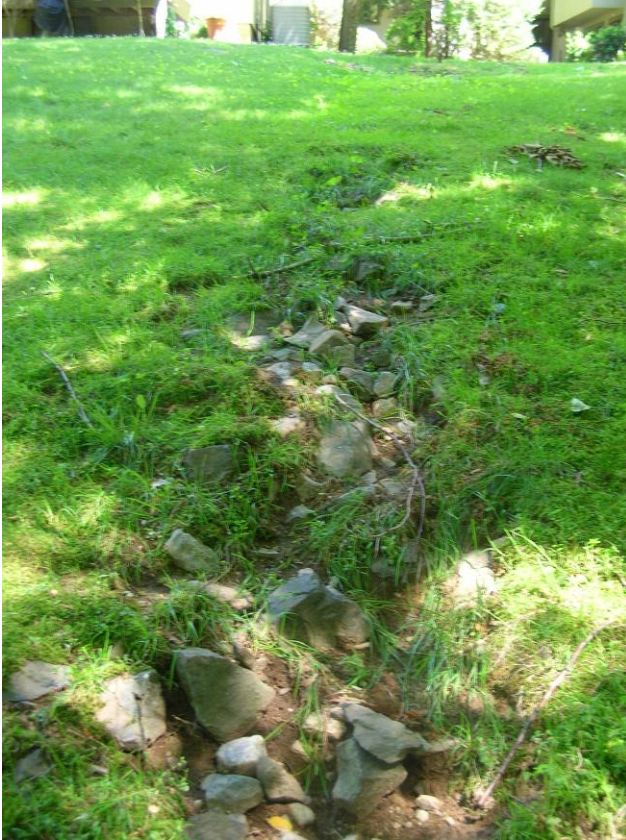
Lawn Area Runoff Eroding Soils
