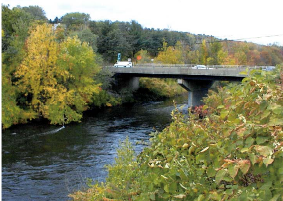
P5 – Huntingdon Avenue Bridge East bank.
