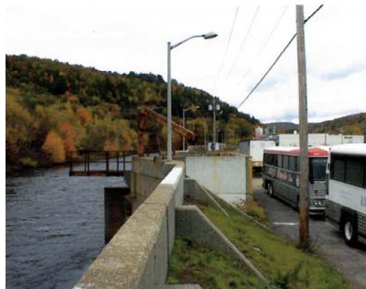
P3 – Looking North
