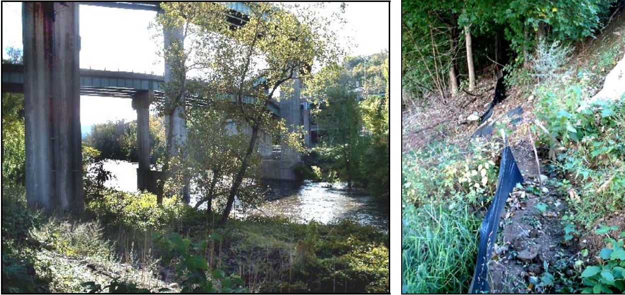
This view under the mixmaster shows lush vegetation and the isolated nature of the river. The view to the right shows the dramatic failure of the erosion control allowing a fan of soil to move downslope to the river. This occurrence is just below the materials recycling operation.
