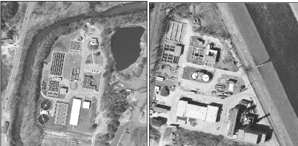
Two Sewage Treatment Facilities: The left hand image is in Harwinton near the top of the watershed and on the right is the facility in Ansonia near the bottom of the basin.
