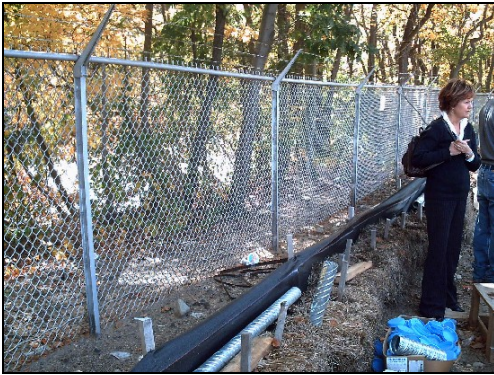
The above photo shows the staked haybale/ silt fence, the chain link fence with barbed wire and a narrow width of surface before the land drops off to the river level. On the right, the Washington Street Bridge is the northern most with the Eagle Street bridge in the center.
