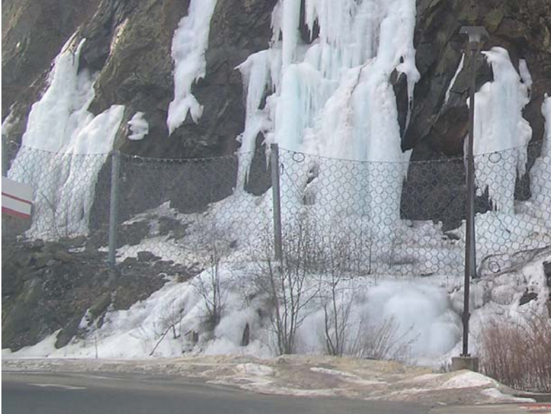
7b. Groundwater seeping from fractures in artificial cuts during winter: spectacular ice-falls result. Note considerable ice coming out onto paved area.
