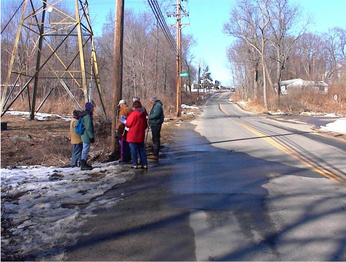
Photo Three: Drainage on Highland Avenue just north of proposed road entrance to project. Drainage here includes stormwater that by passes factory driveway (up past the street sign) as shown in Photo Two . Note that there does appear to be some erosion along the edge of the pavement.
