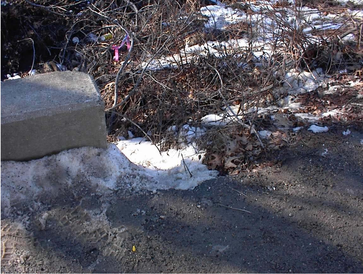
Photo Four: (Point A on Figure Four). Note sediment on pavement in foreground, eroded soil and damaged pavement at culvert headwall (Photo looks west).
