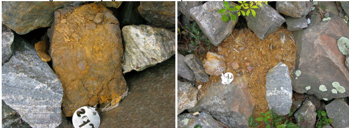
Figure 3. Fragments of Brimfield Schist that are part of the dam for Lower Bolton Lake. They contain iron sulfide minerals that weather by dissolving and releasing iron oxide and sulfuric acid to the environment. Iron oxide is precipitated almost immediately in an oxidizing environment. Note on the right that what was originally a rock fragment is now rubble. Disc on key-chain in both images is 2 inches in diameter.
